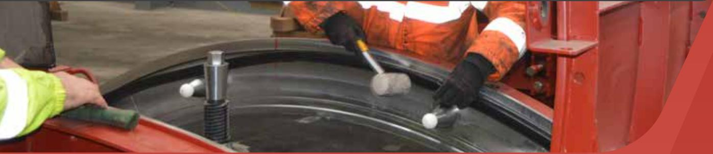
Cast-in gaskets are integrated with the segment during the casting process as opposed to being glued into a pre-made groove once the segments have been cast. Cast-in gaskets are cleaner to work with and are rapidly becoming the preferred choice of designers and pre-casters by eliminating the need for applying adhesive while providing cost and time savings by removing extra installation processes.
