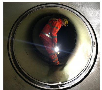
Inspection of the VIP-Weco - post installation
